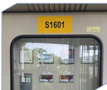
Frequency adjustment for Area 16 50HP exhaust fan S1601
