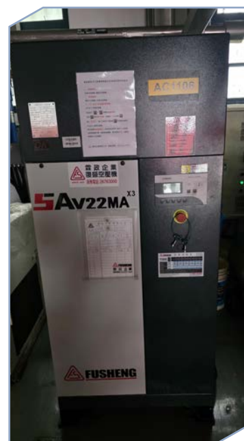
Replace old 15HP air compressors in Zone 13 with new ones
